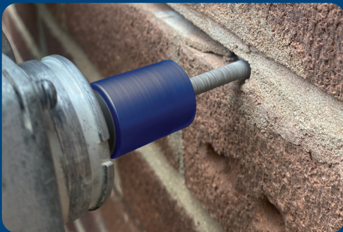
MORTAR RAKING GORES IN ACTION
