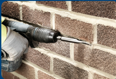
MORTAR RAKING CHISEL IN ACTION
